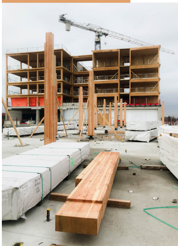
A Mass Timber building under construction in Toronto, Ontario. Source: Pilot Projects, 2022.
