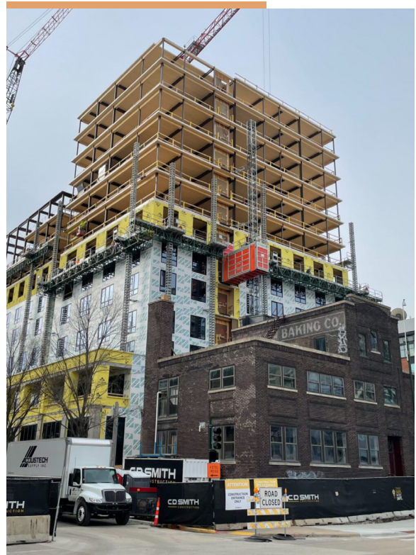
The Bakers Place project is a 14-story building consisting of a 3-story concrete podium and 11 stories of mass timber-steel hybrid construction with a primarily residential program above it. Source: The Neutral Project and Michael Green Architecture.
